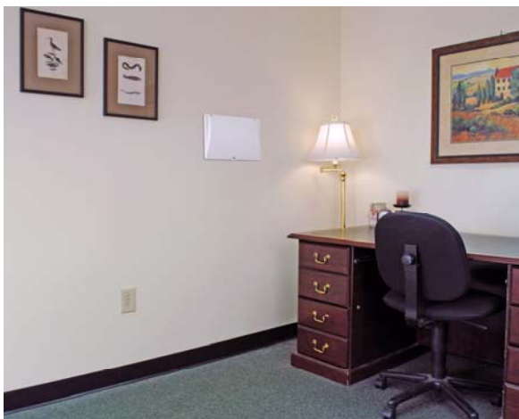
Oberon's Wireless Router Box recessed in wall
